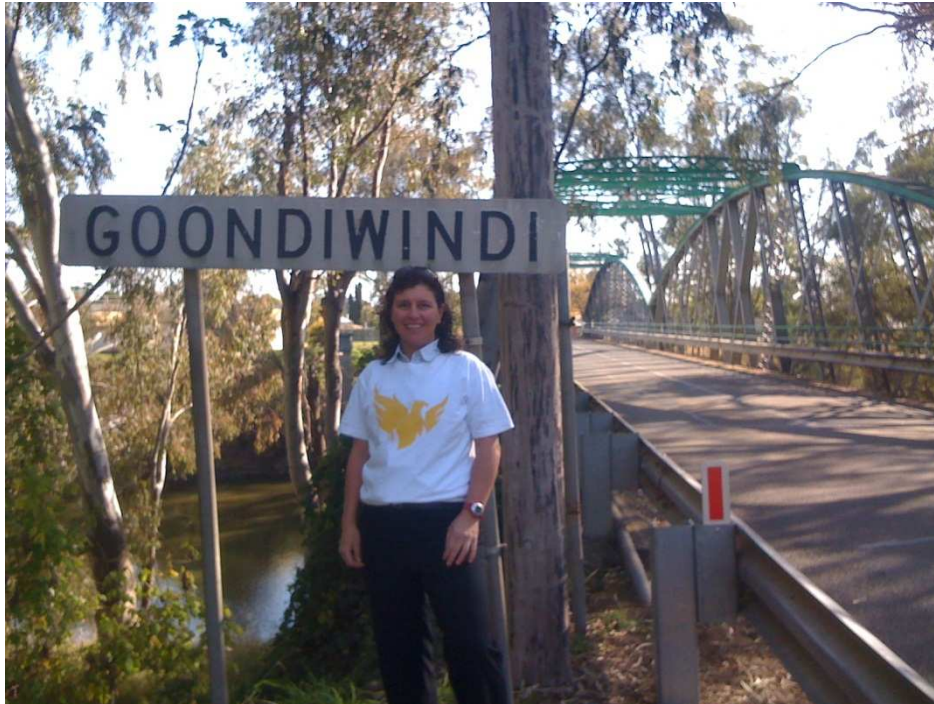
Study 7 Figure 5 The levee bank at Goondiwindi protects the town from the Macintyre River
