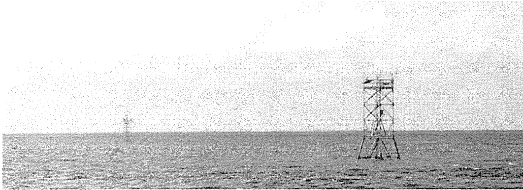
Figure 14: Davies Reef: the old tower (left) will be decommissioned later this year. The newly designed tower (right)
