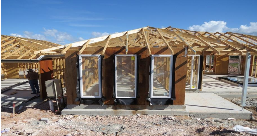
Figure 2 Contemporary house under construction
