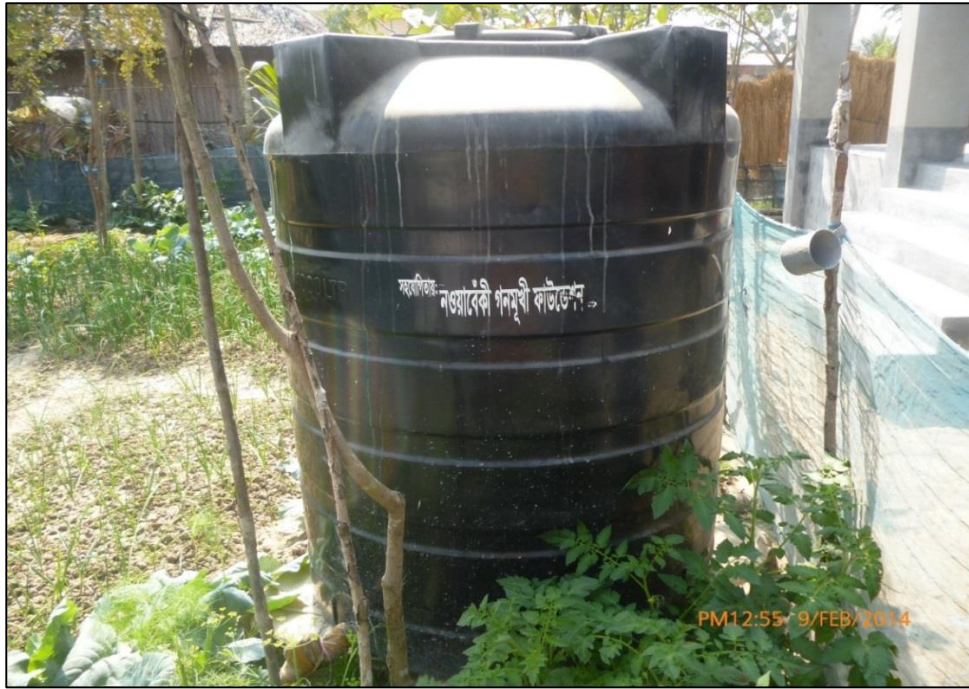
Figure 7-3: Water tank to reserve rain water to be used for the whole year in Gabura
