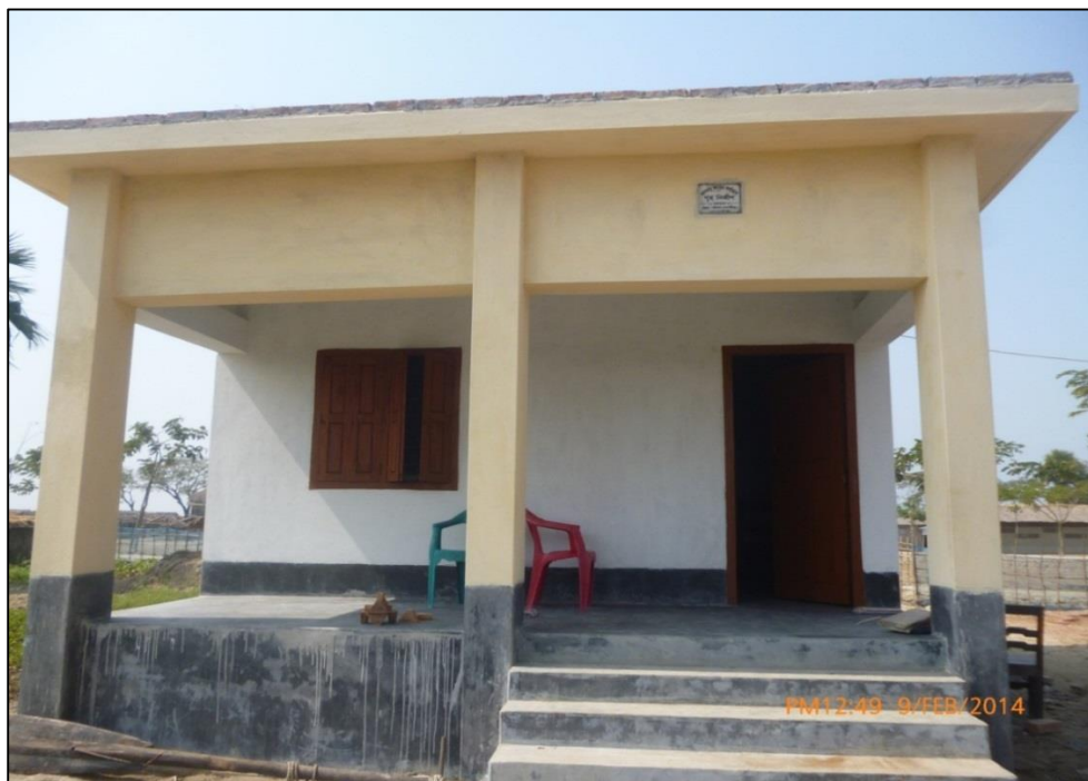
Figure 7-2: A one room house built for a poor family in Gabura
