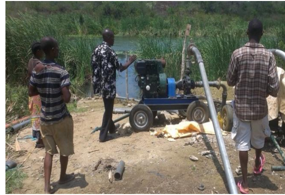
Plate 4.4: Dam with diesel operated water pump
