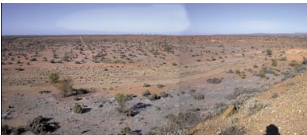
Fig. 5: View from the top of the capped Main Tailings Dam (MTD) towards the SE. Variable amounts of wind-blown tailings are present in local topsoils due to wind deflation prior to capping of the MTD.
